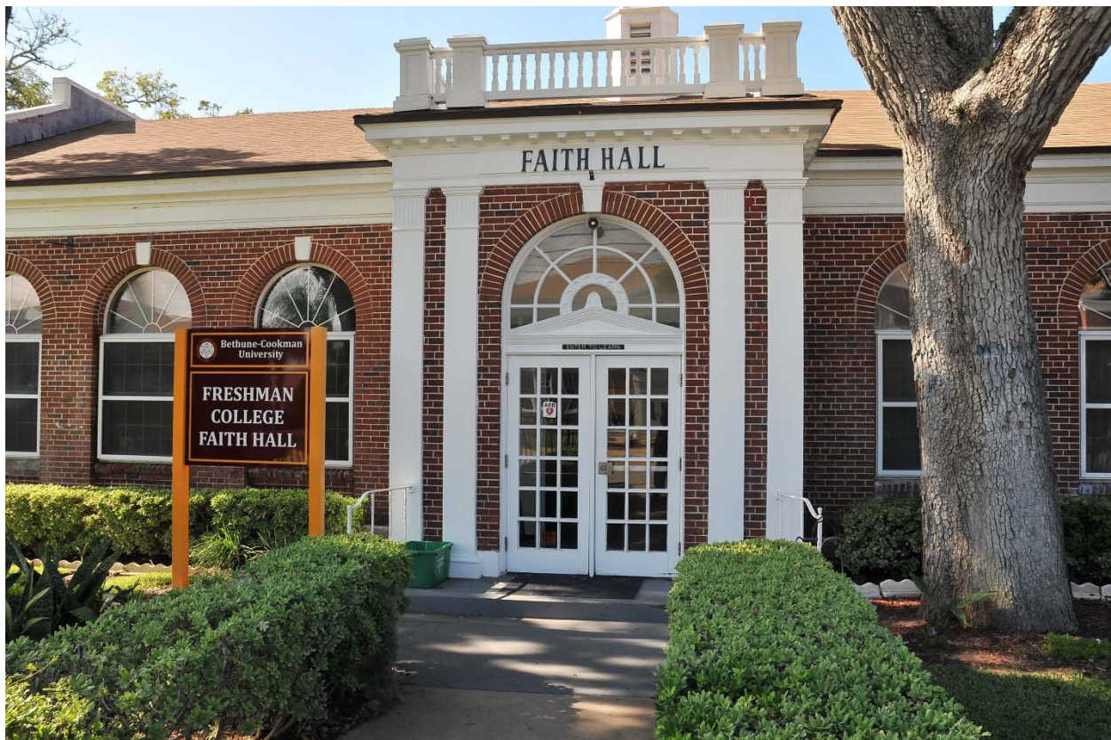
Historical Faith Hall; Administrative Offices for Freshman College
